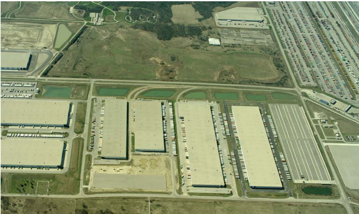
Figure 4.B.10b. Center Point Distribution Center, Elwood, Illinois at BNSF Logistics Park-Chicago.
