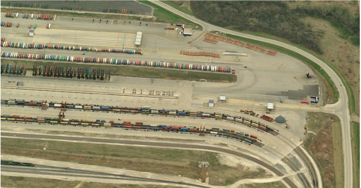
Figure 4.B.10a. Elwood, Illinois BNSF Logistics Park-Chicago Interchange Hub Exit
