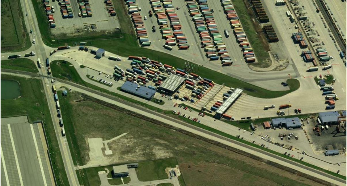
Figure 4.B.9. Elwood, Illinois BNSF Logistics Park-Chicago Interchange Hub Entrance
